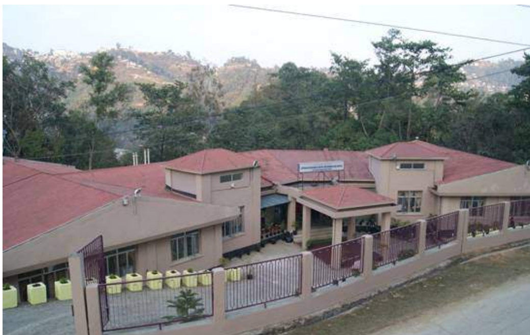
Figure 4: Office Building of ICFRE-BRC, Aizawl, Mizoram
