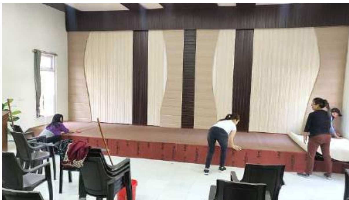
Conference Hall Renovation – Stage Carpet Installation
