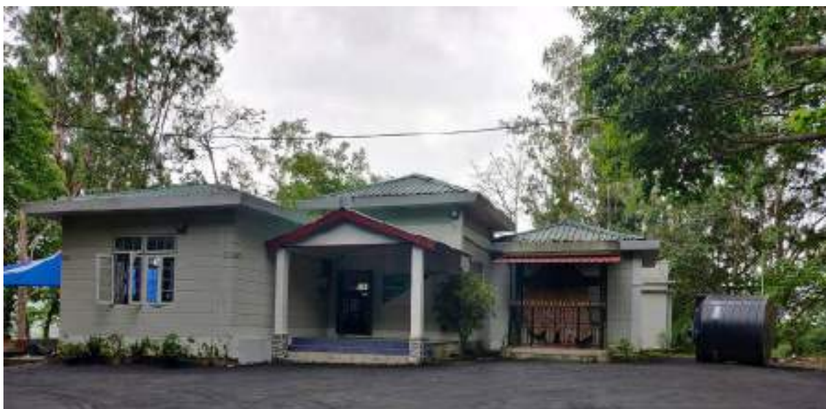
Black Topping of Principal Courtyard and Internal Road within FTS
