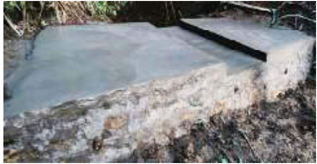
Masonry Check Dam
