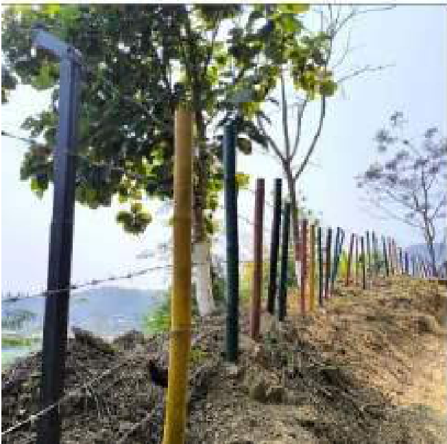
Barbed Wire fencing using Angle Iron Post with R.C.C Foundation
