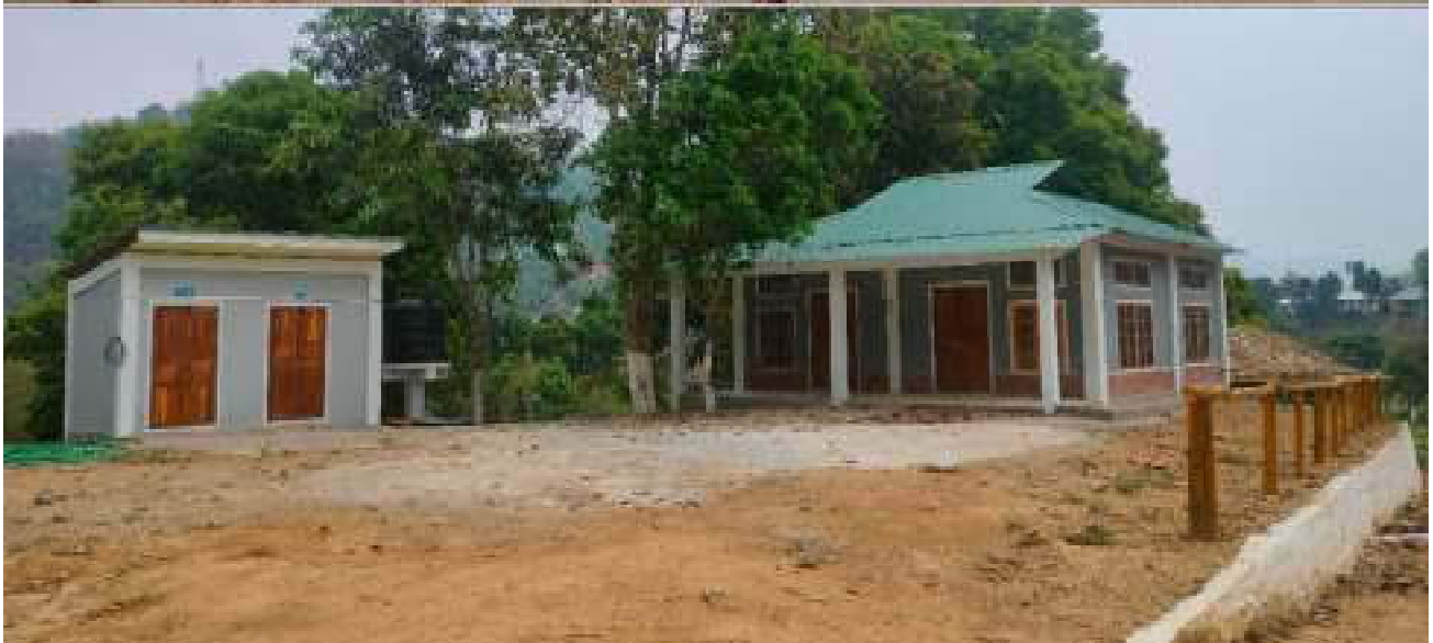
Construction of Nature Interpretation Centre
