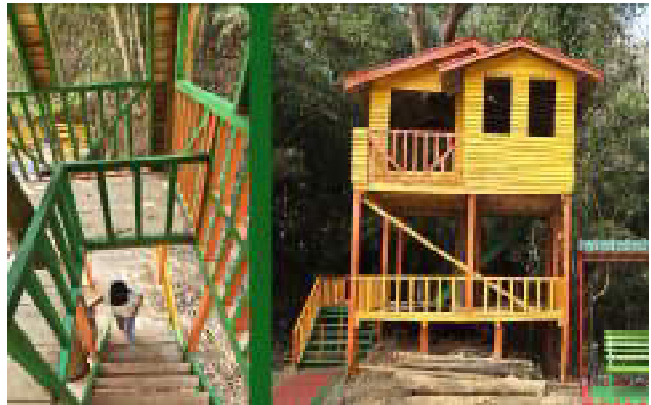
Construction of Tree House with deck for bird watching
