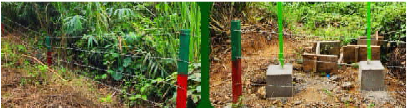
Providing and fixing of Chain Link/Barbed Wire fencing using Angle Iron Post and Barbed Wire
