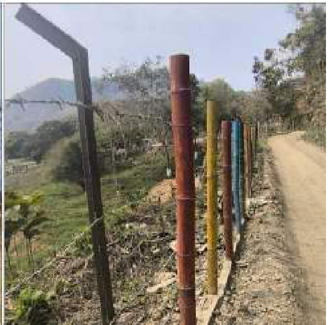
Barbed Wire fencing using Angle Iron Post with R.C.C Foundation
