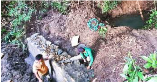
Masonry Check Dam
