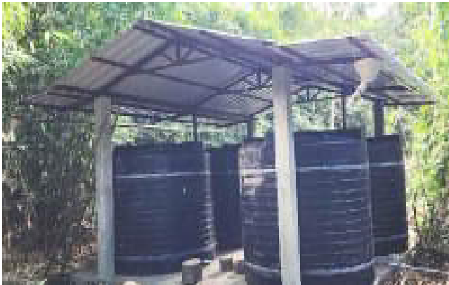
Rain water harvesting (RCC structure and foundation) with roof truss 20000 ltrs.
