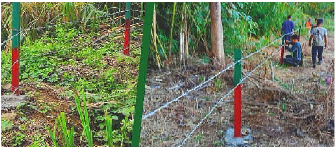
Robust Angle iron post with solid foundation
