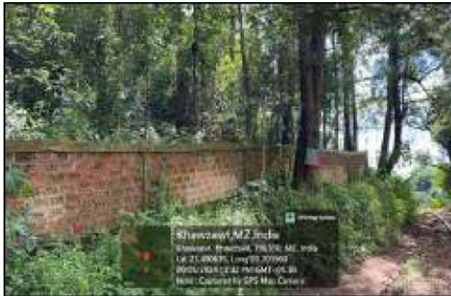
Brick walled fencing with angle iron post
