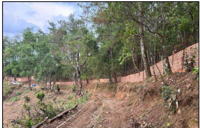
Brick walled fencing with angle iron post
