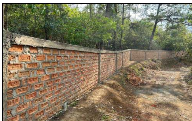
Brick walled fencing with Angle iron posts
