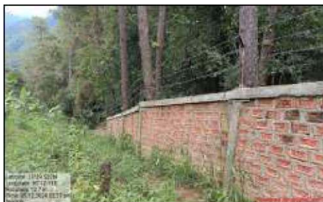
Brick walled fencing with Angle iron posts
